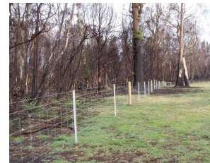
Pine post in-lines and strainer assemblies with hinge joint
